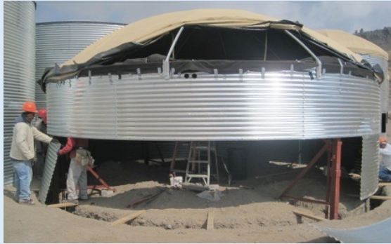
Steel frame construction
